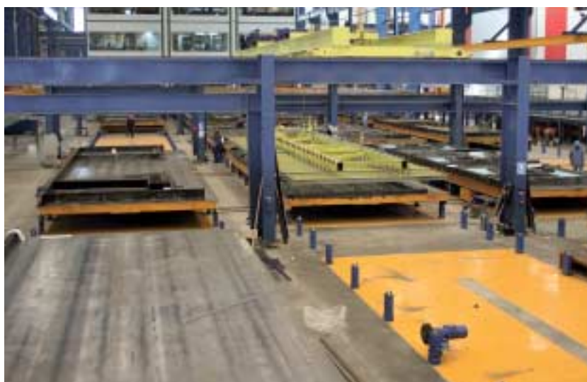
Fig. 9 The individual manufactured reinforcing mesh is lifted on the prepared pallet.
