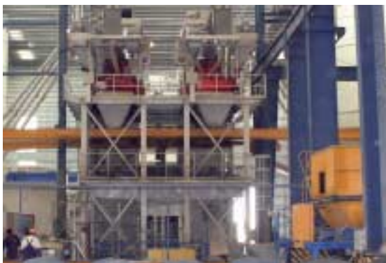
Fig. 3 The mixing plant and the silos for cement and aggregates storage.
