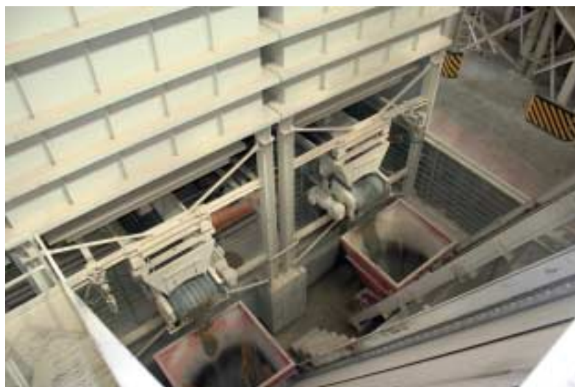
Fig. 1 Feeder skip hoists for the mixers.
