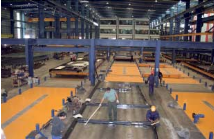
Fig. 7 Working steps before concreting are made on three parallel lines. The fourth line (rightmost in the figure) is used for the preparation of the second concreting process for sandwich panels.
