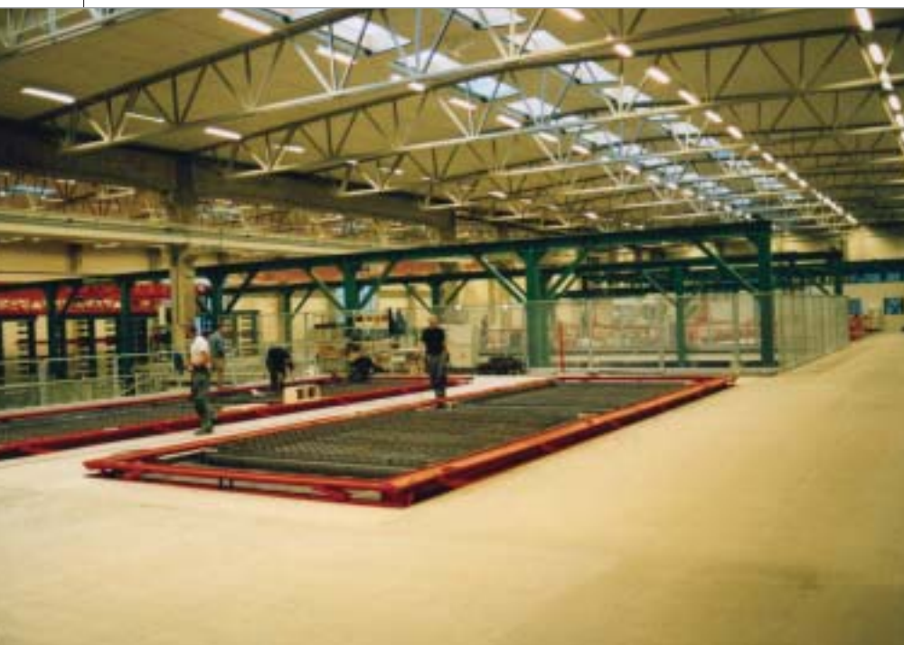
Reinforcement extension working area
