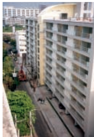
Bilder 1, 2. Appartementhäuser in Typ Condo Figs. 1, 2. Apartment buildings of Type Condo
