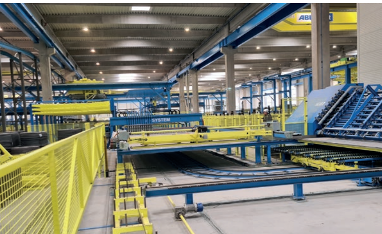
Mesh welding plant
