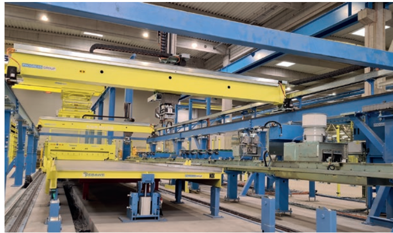
Shuttering and demoulding robots precast floor slab plant
