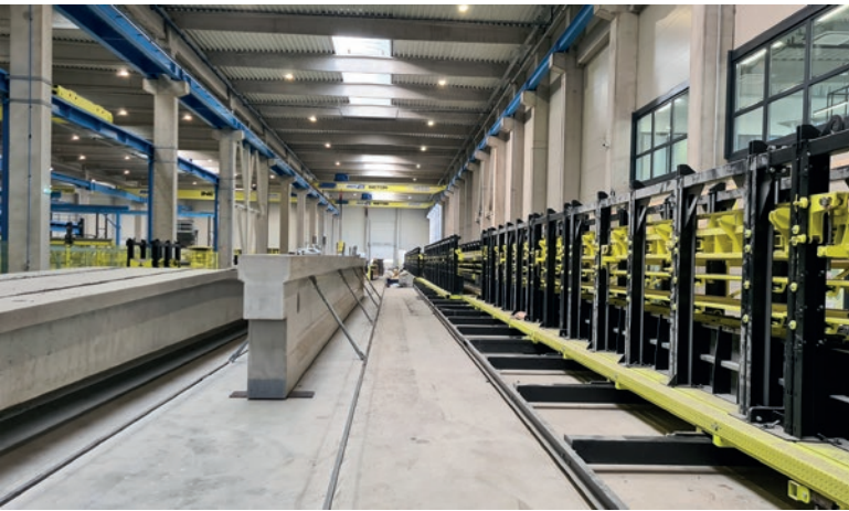
Prestressed concrete hall
