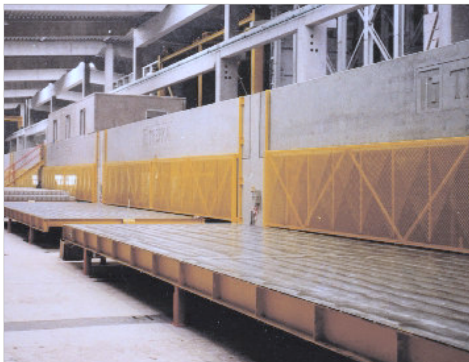
Moulding and reinforcement area
