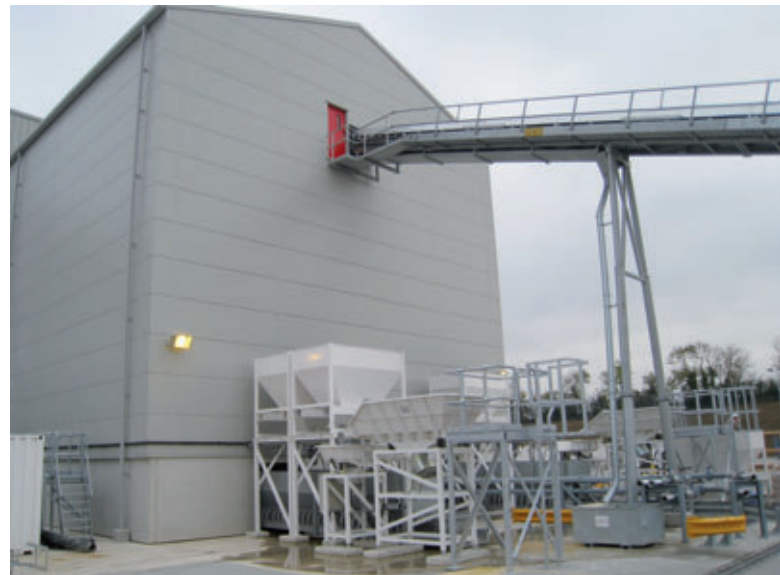
Fig. 36: Skako Concrete Batching Plant
