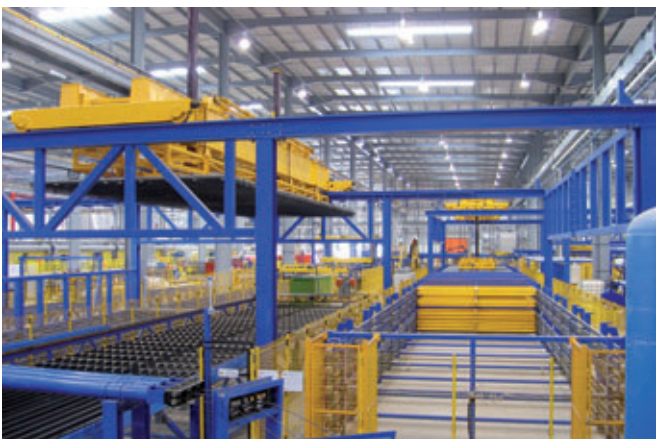
Fig. 30: Mesh Crane and Buffer Store
