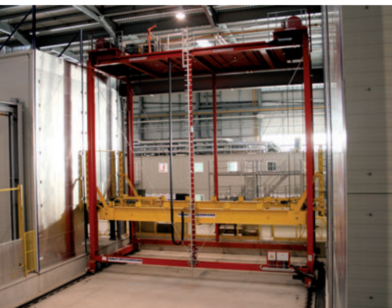
Fig. 21a: BSC Rack Operator
