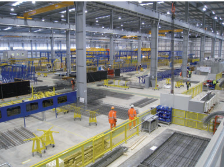
Fig. 35: Cage Assembly Area
