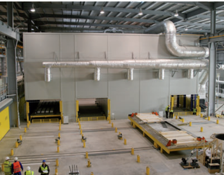
Fig. 20: Concrete Pouring and Finishing Area, Curing Racks
