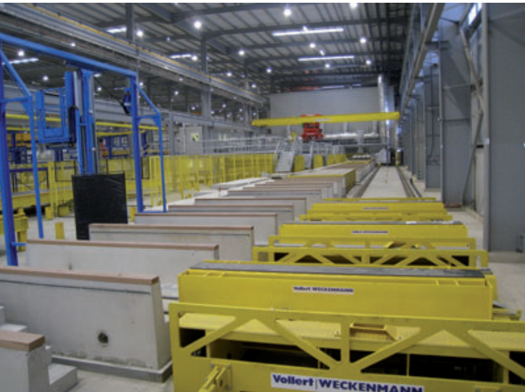
Fig. 15: Unloading Area and Run-off Truck
