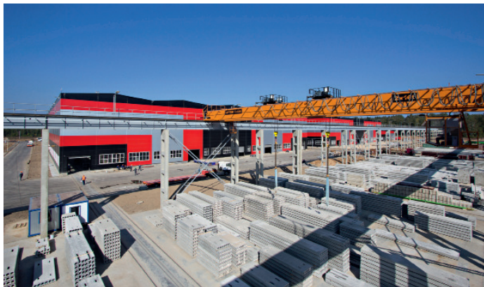
View from the storage area on one of the production facilities of the precast plant DSK Grad in Kotovo in the greater Moscow area
