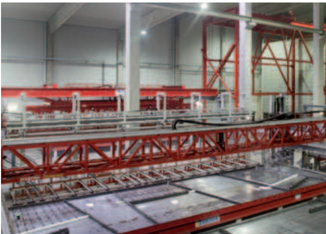
Reinforcement installation by the reinforcement robot
