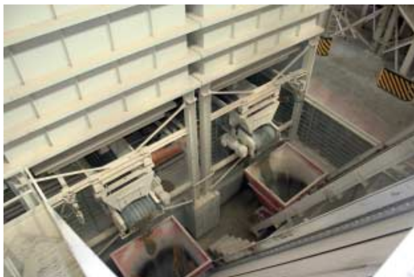
Fig. 1 Feeder skip hoists for the mixers.
