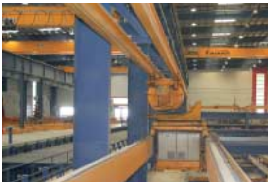
Fig. 4 Three dump skips transport the fresh concrete to the different production lines.
