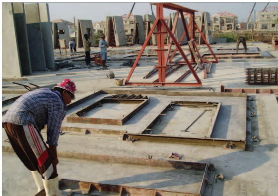
Casting Yard Preuksa
