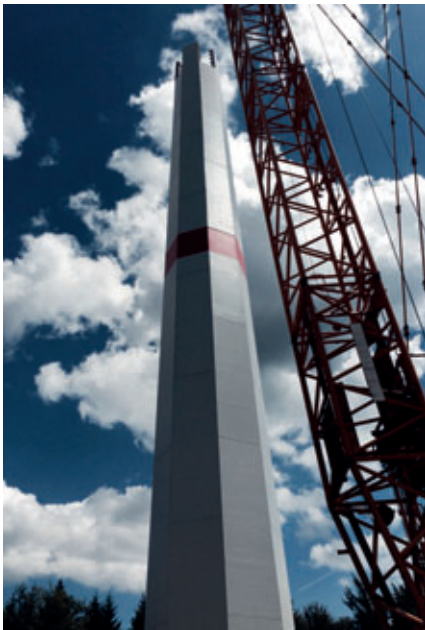
Patented Ventur hybrid tower for wind turbines
