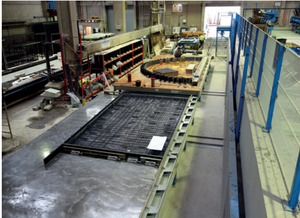
Fig. 5: Shuttering and reinforcing stations for solid/sandwich walls and custom elements
